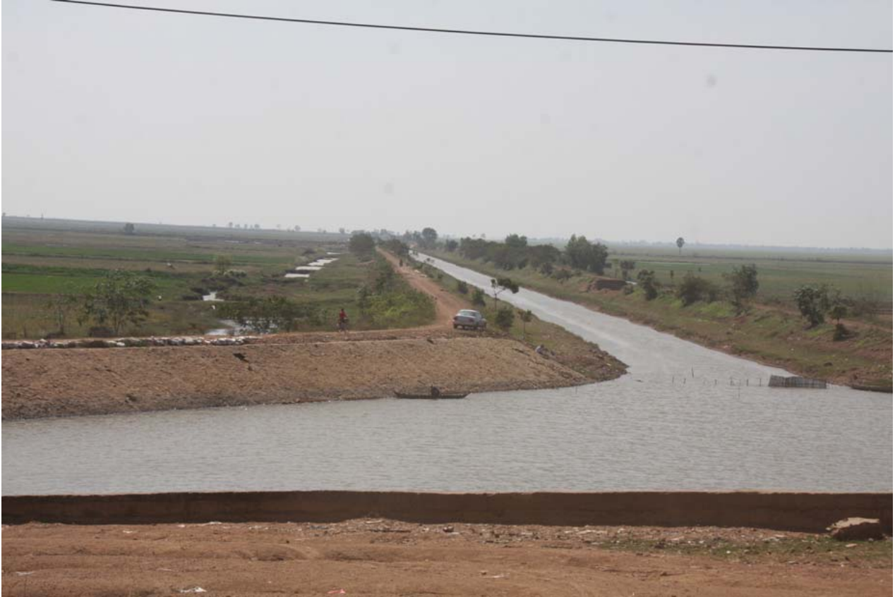
Trapeang Thma Dam, December 2013 (Source: Documentation Center of Cambodia) 401
